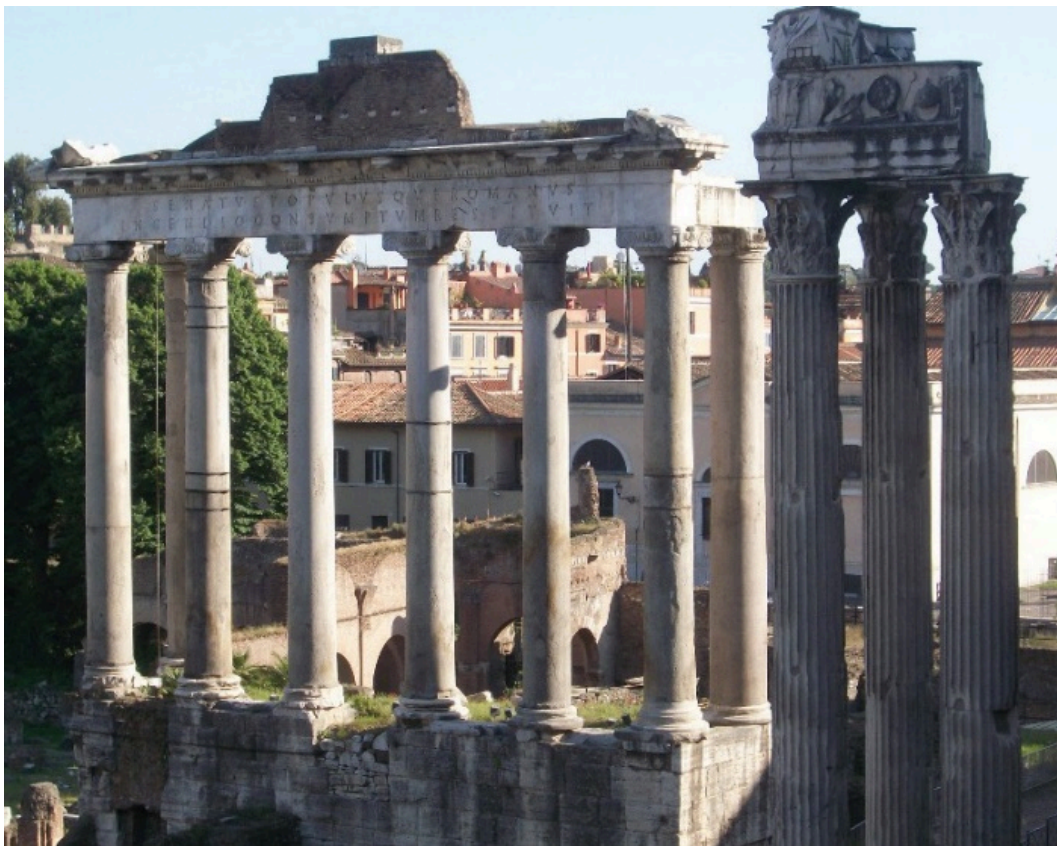
Figure 8.15 | The Roman Forum. Why did the Romans use so many vertical columns to hold up the one horizontal beam? If the horizontal beam spanned a long distance without support, it would buckle under its own weight. This beam is experiencing tensional stress, and rocks have very little strength when exposed to such stress. Source: Randa Harris (2015) CC BY-SA 3.0 view source
